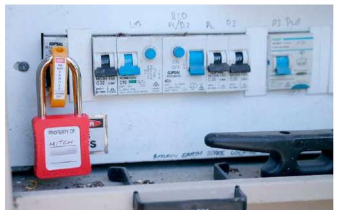
Image 11: Example of main electrical switch with lock
