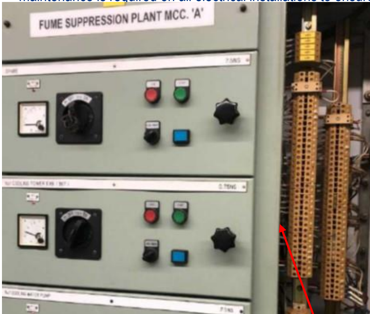
The MCC tier showing the two cells and the adjacent cable launder tier. Control wire was hidden behind this flange.
