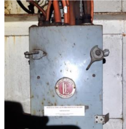
The supply fuseboard with all the cables top entry. Below the internal bottom of the fuseboard with moisture and rust evident.
