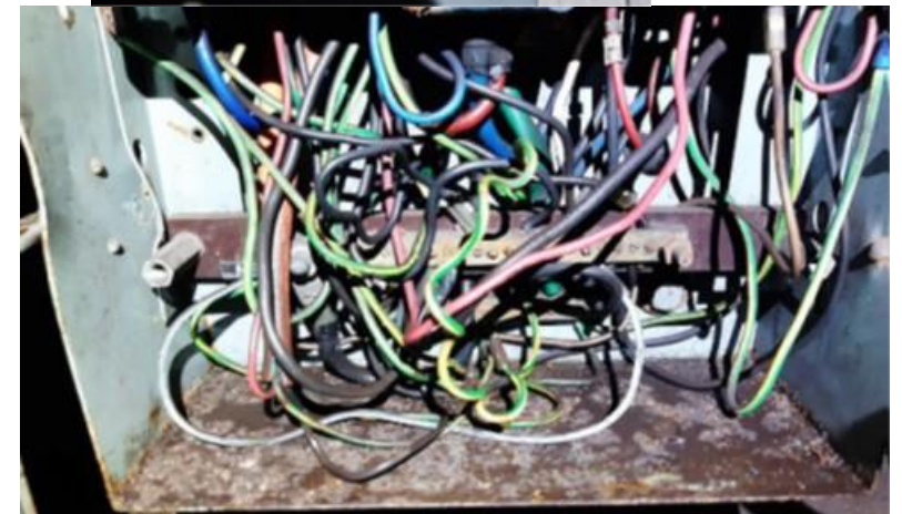
The supply fuseboard with all the cables top entry. Below the internal bottom of the fuseboard with moisture and rust evident.
