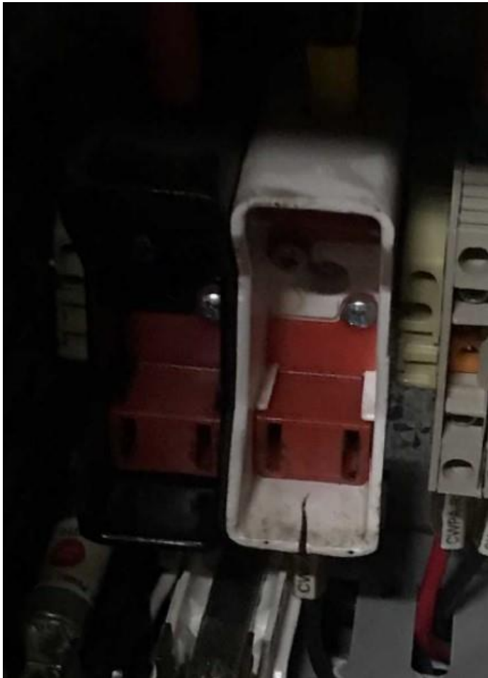
One of the neutral link holders found in the MCC with signs of cracking as opposed to the red spot fuse holder which is in good working order
