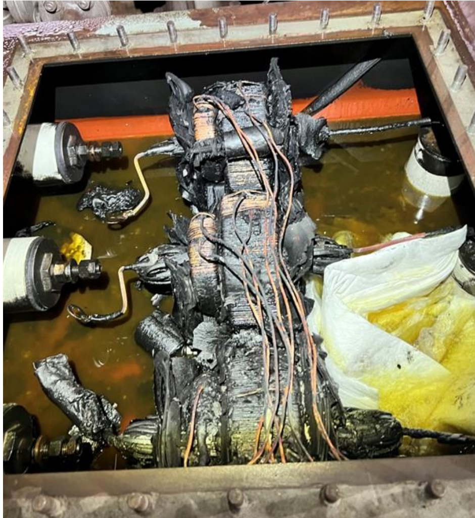
Inside the link box after the fire, with the cabling and CTs destroyed
