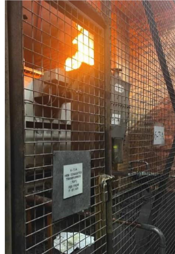
The 33kV to 1200V drive transformer enclosure, with fire coming from the link box on the 33kV side
