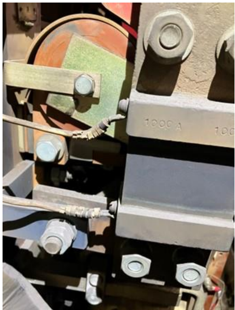
The DC shunt rated at 1000amps
