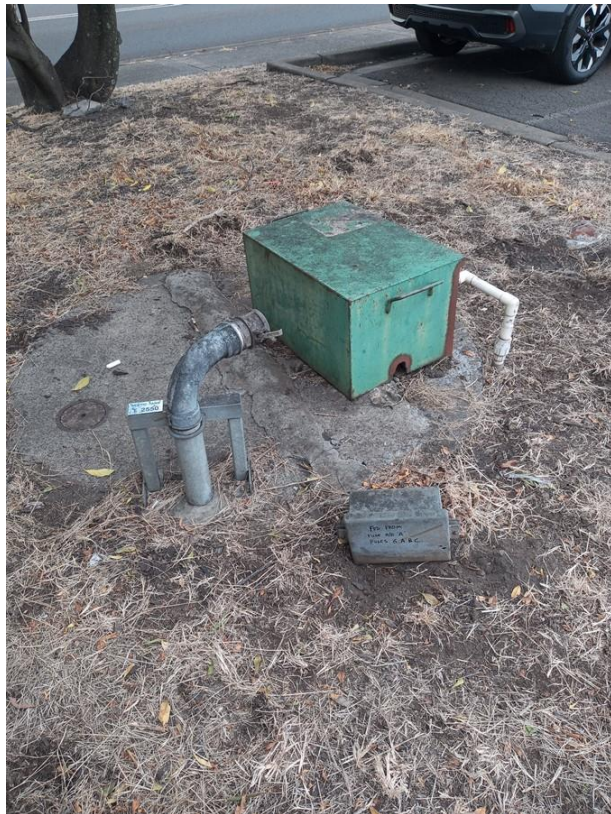
The septic tank area
