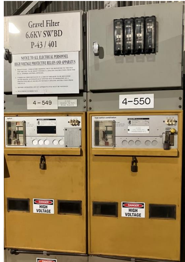
6.6kV Circuit Breakers and contacts inside
